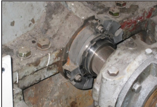
The Chesterton 442 Split Seal can be installed without dismantling the pump.
