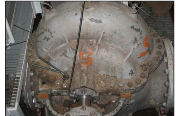
Chesterton 442 with Plan 11 Discharge Recirculation.
